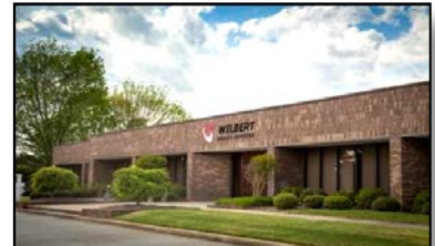
Easley SC Facility (ESC)
