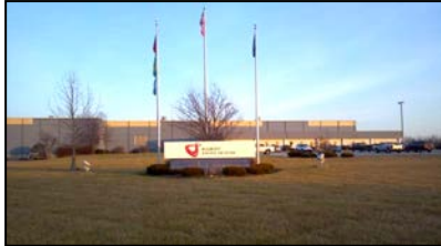
Lebanon KY Facility (LKY)
